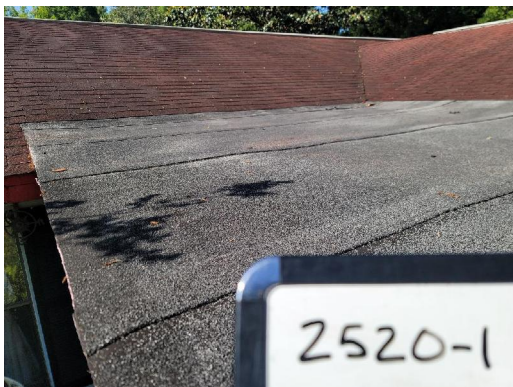
2520-1 Asphalt Shingle/Membrane Exterior Front Porch Roof
